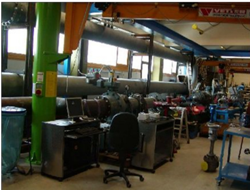
Test station (2-way pipe test loop) approved by PTB METRA Energie-Messtechnik Speyer
